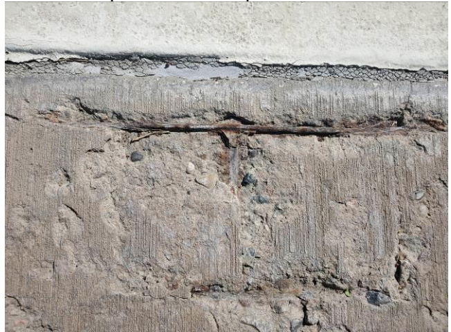
Photo 4: Exposed rebar in pool deck
