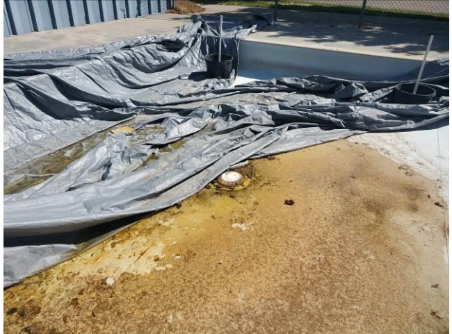
Photo 8: Single wading pool main drain
