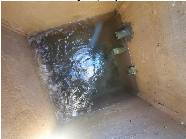
Photo 3: Limited surge capacity
