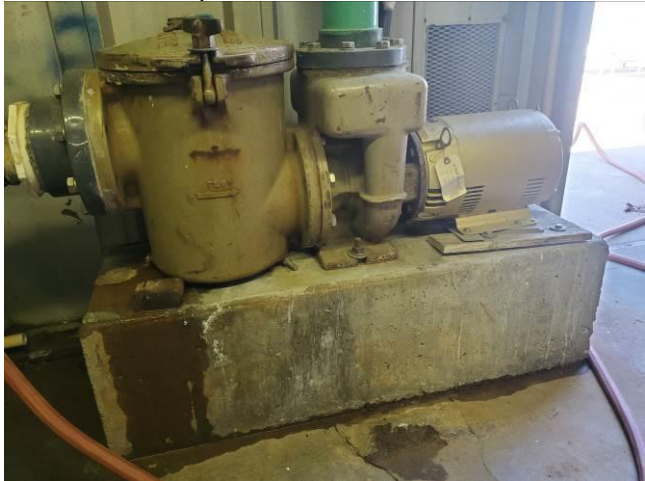
Photo 11: Pump above water level
